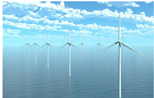
The deployment of wind power generation is expected to expand toward the realization of a carbon-neutral society.
